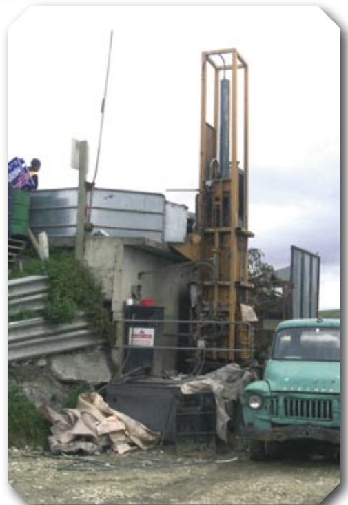
Waste management - recovery shed (above) and the refuse press (below)
