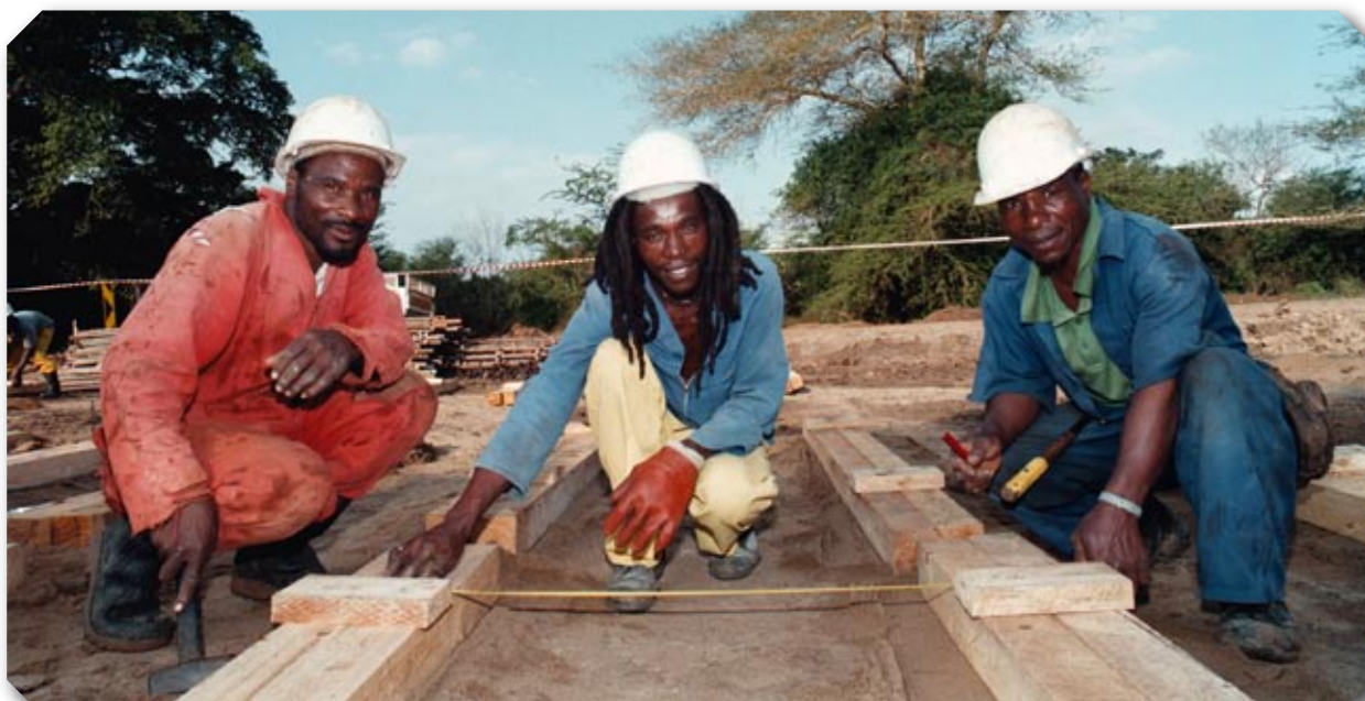
Tourism and local communities benefit from bridge construction Photo: Great St Lucia Wetlands Park
