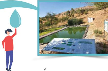
When the channel of the constructed wetland receives the pretreated wastewater, aquatic plants release oxygen from their rhizomes, which stimulates both the decomposition of organic matter and the growth of nitrifying bacteria. Nitrifying bacteria then convert ammonia to nitrate. The nitrate formed diffuses or percolates through to the oxygen poor zones where it will be removed from the system by denitrification.
