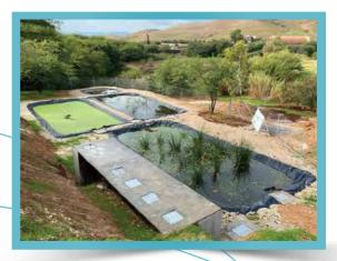
A wetland is an ecosystem that is permanently or seasonally flooded by water. A constructed wetland is a man-made structure that is designed to mimic the natural functions of wetlands. The constructed wetland consists of constructed channels with planted filter beds that provide space for waste water treatment by biological processes. These planted filter beds are commonly made of gravel or sand.
